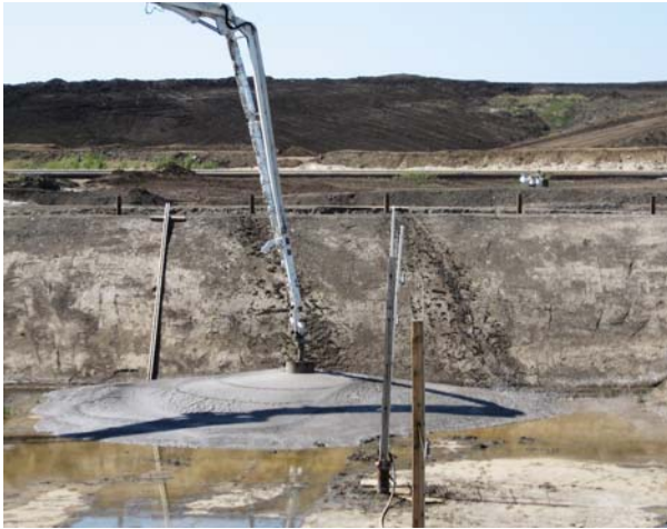
Figure 3. Start of NST deposition in Cell 5
