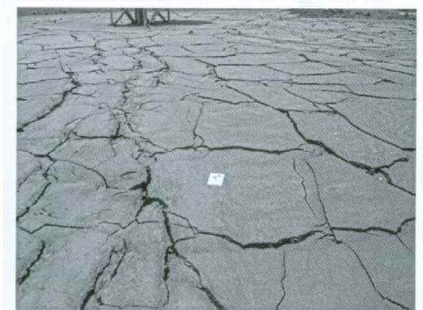
Figure 7. Desiccation and cracking of the deposited TT (paste) after 5 days (Lord et al., 2002).
