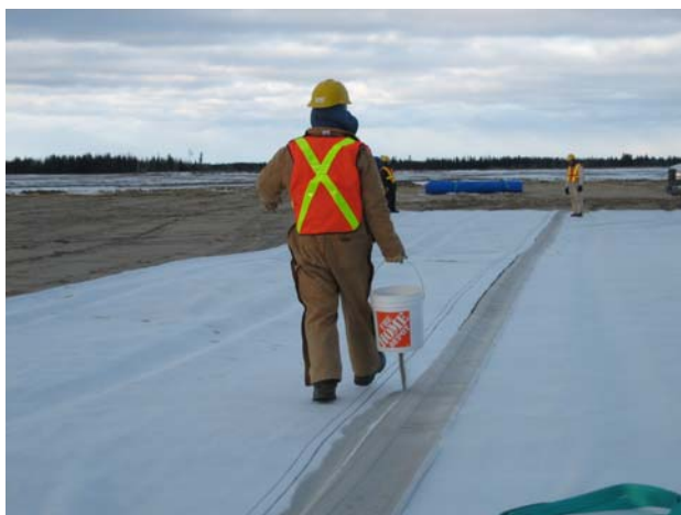
Figure 4. Spreading of the loose bentonite between GCL sheets.
