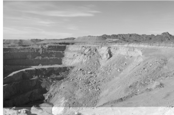
Figure 2. Photograph of the Progression of the May 2008 Slope Failure, Observed November 2008
