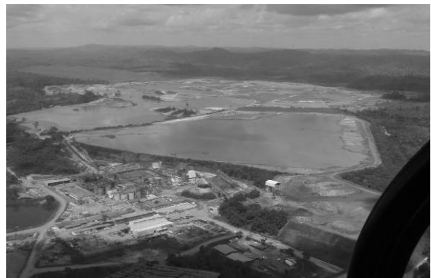
Figure 1. Tailings disposal facility at Bogoso
