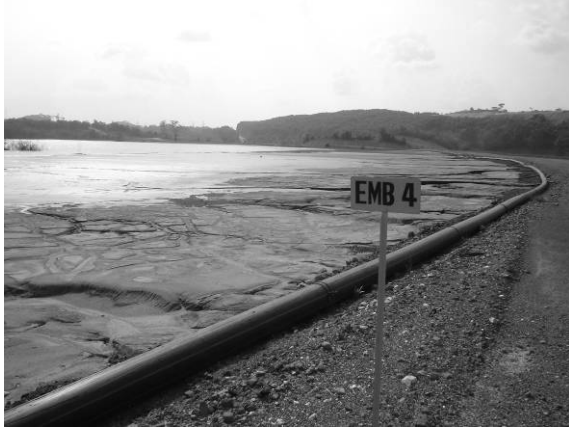
Figure 2. Bogoso/Prestea Tailings Disposal Facility showing spigots and beach
