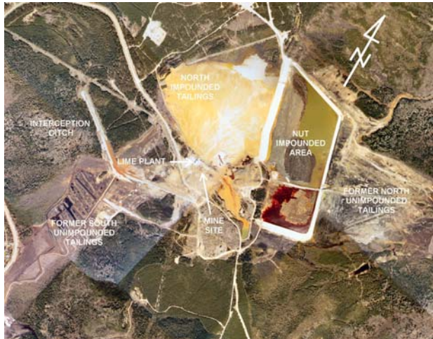
Figure 1. Aerial view of the abandoned Kam Kotia Mine site prior to implementation of a multi-staged rehabilitation program.
