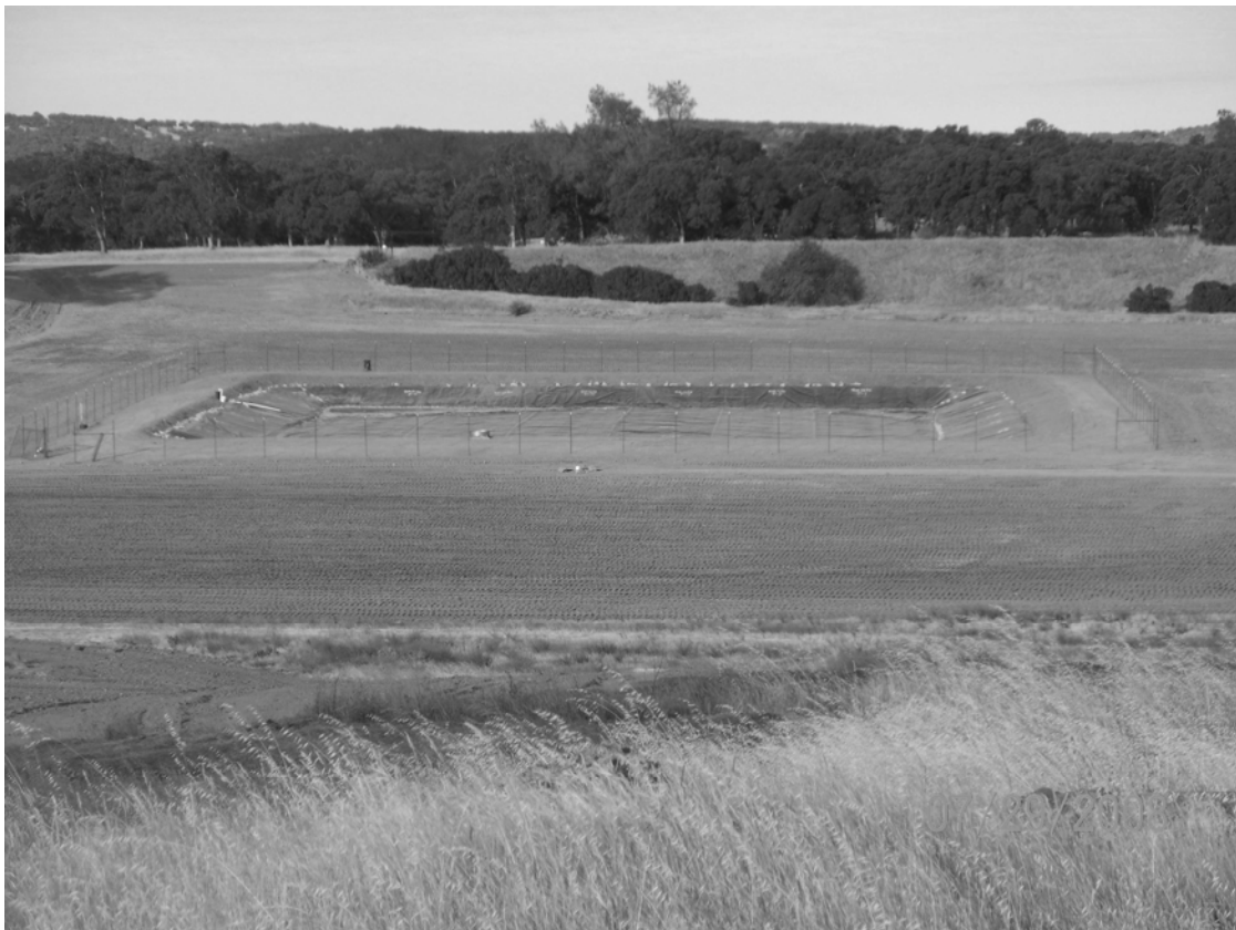
Figure 6. Closed PWP with Evaporation Pond (September 2008)
