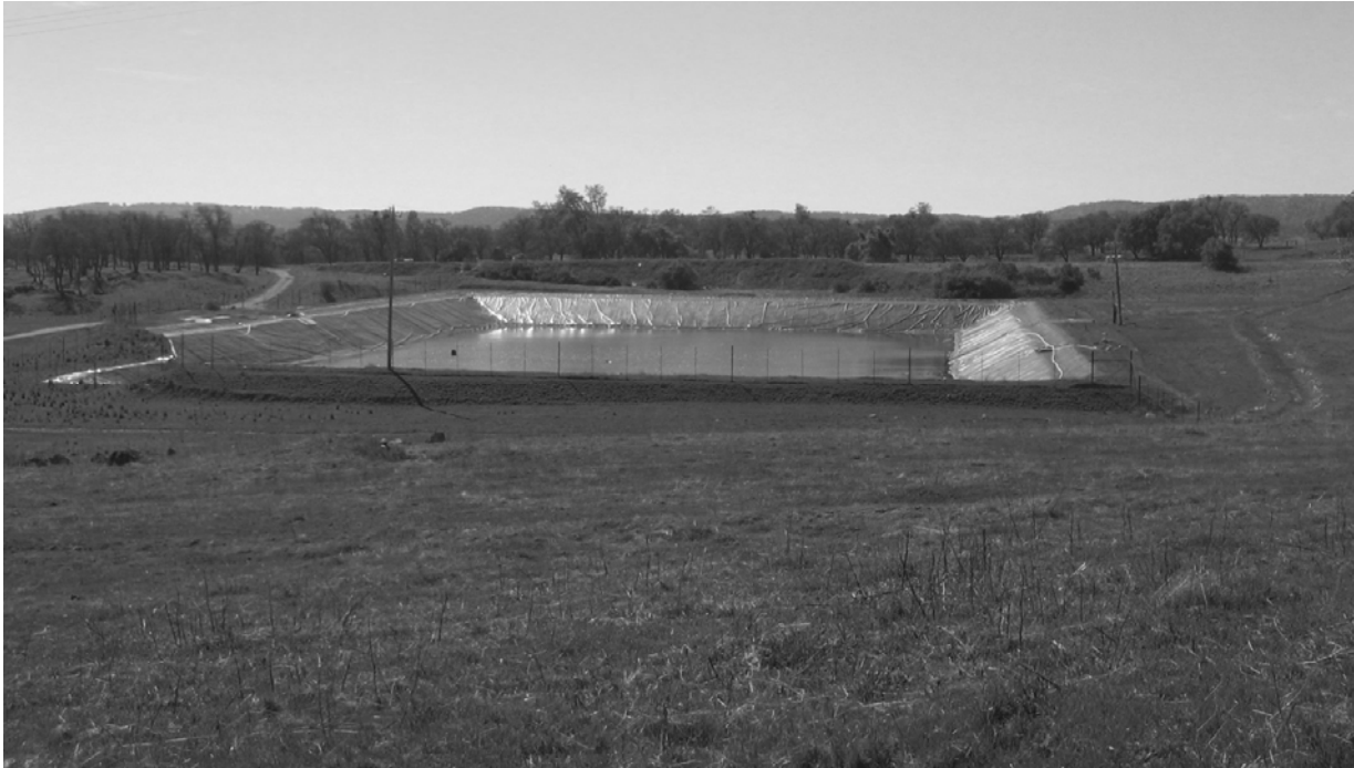
Figure 1. PWP Prior to Construction (March 2007)
