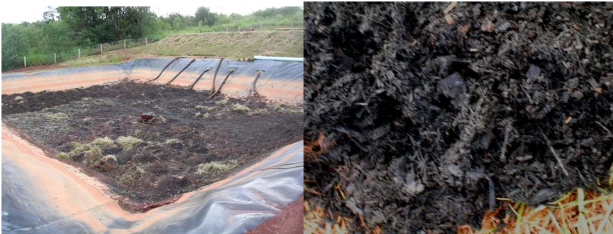
Figure 8. The ZVI/organic reactor being filled and the substrate just below the surface after six months of operation.
