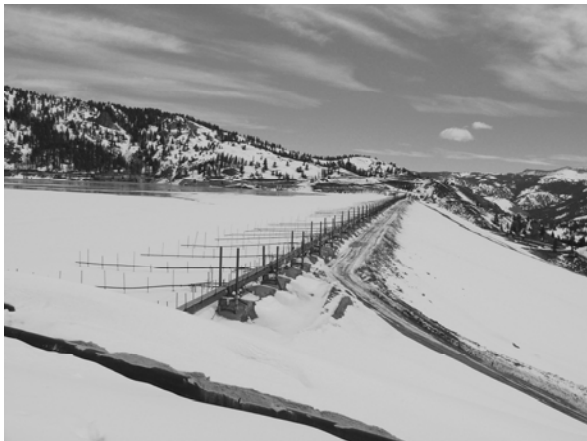
Figure 1. Cycloned sand dam construction.
