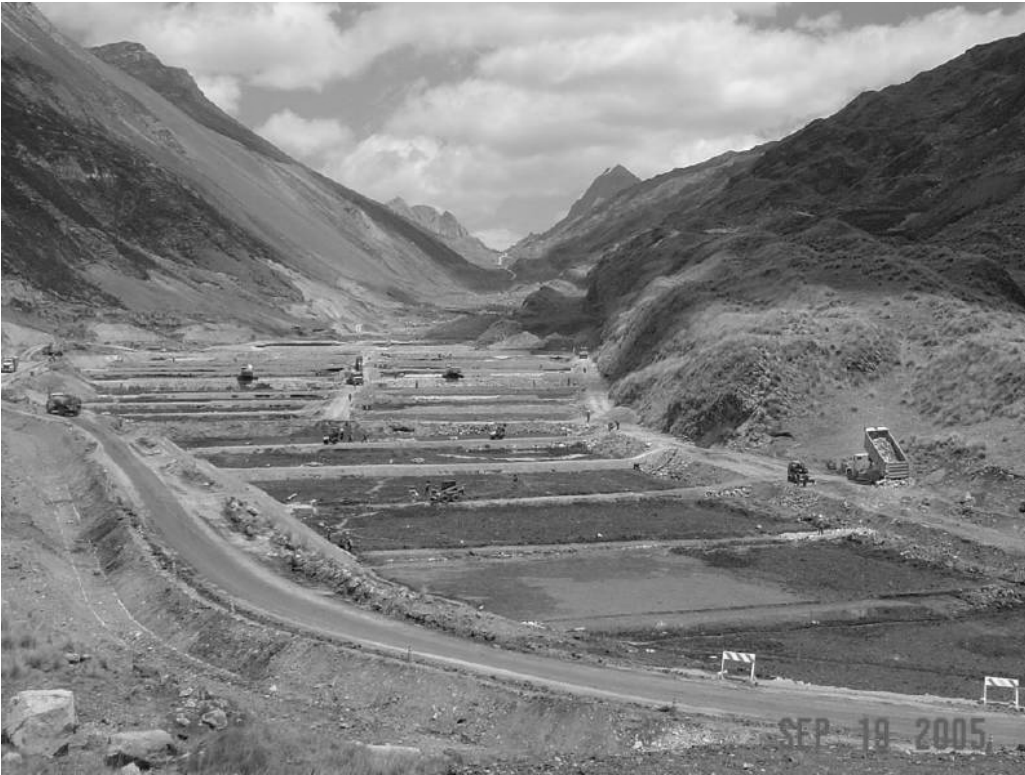
Figure 3. Tucush Valley water treatment system during construction.
