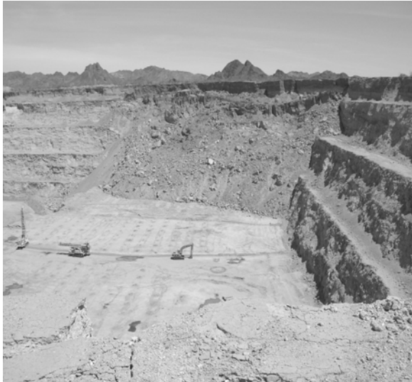
Figure 1. Photograph of the May 11, 2008 Slope Failure of the North Pit Wall
