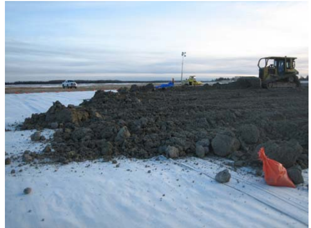
Figure 5. Clay being applied over the GCL.
